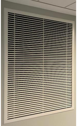
Smoke Control Damper
